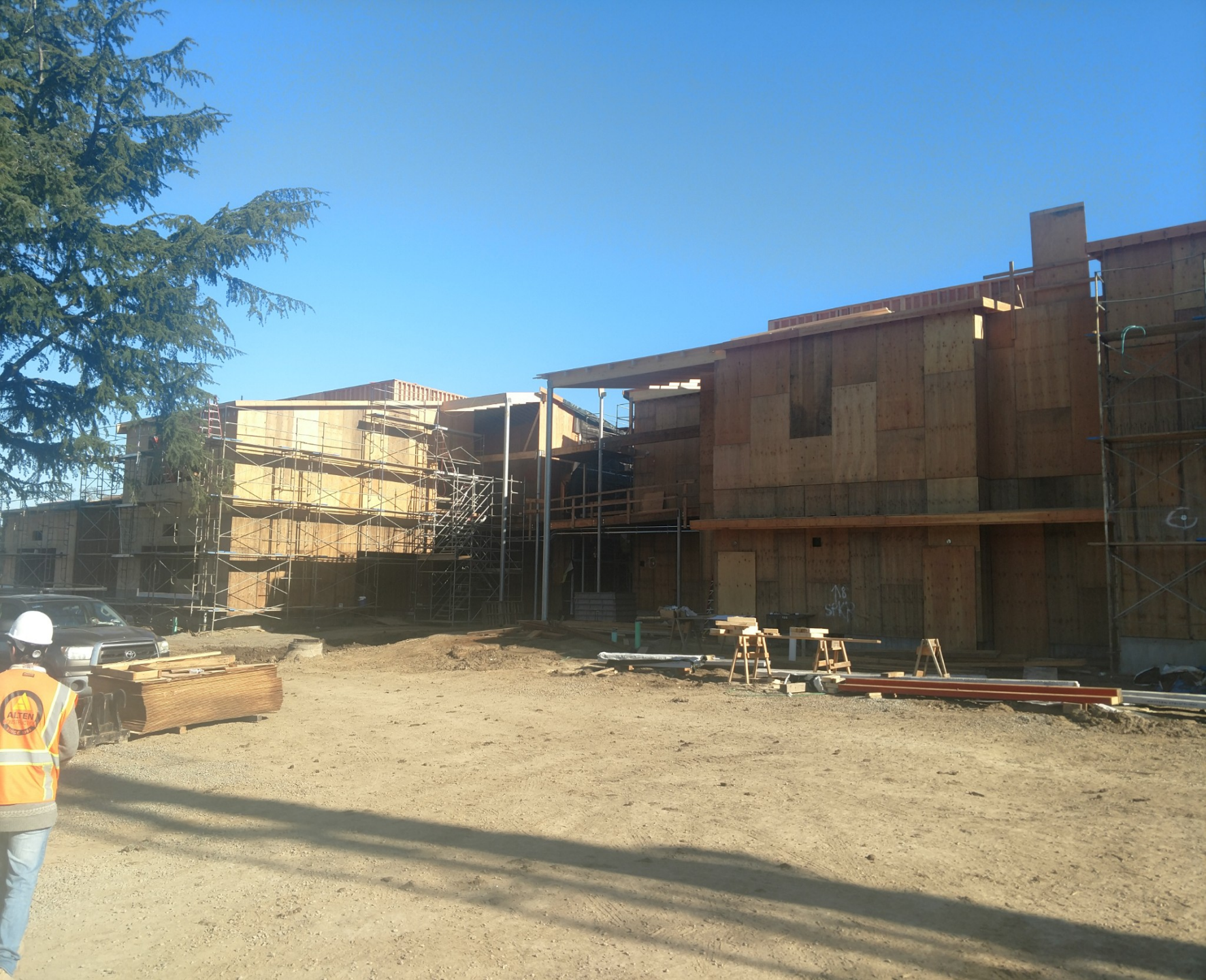
VV 2 Story Classroom Building
